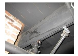
X.7 \$\$ Flashing is installed between the left deck framing and flooring but does not have a drip cap to help prevent water from being redirected back across the bottom of the flashing towards the building. There is also no flashing installed between the bottom of the left deck floor frame and wall. There may be concealed damage.
