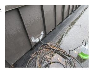
R.5 \$\$ Flashing sleeve is too large for one of the sewer vent pipesand had to be filled with sealant.
