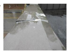
R.11 \$\$ One or more lower pieces of metal coping not extend up behind vertical pieces. See left photo. Right photo shows correct flashing of this coping.
