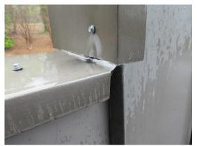
R.12 \$\$ Flashing is missing at the front left corner where metal meets stucco on the parapet wall.
