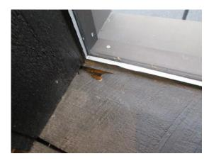
X.4 \$\$\$ Puddles on the basement floor and wet wall brick and wall covering, especially at the left side, indicate continued water seepage into this finished basement area. See examples in photos. Consult a professional basement drying company for evaluation and repair.
