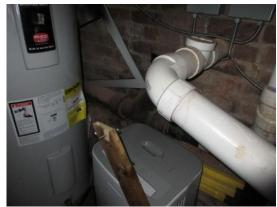
P.d The pans and/or drains installed beneath the water heaters were not tested for functional flow.
