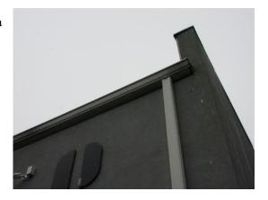
Stucco has cracked/separated in areas, especially at the left rear corner and a front left window area.
