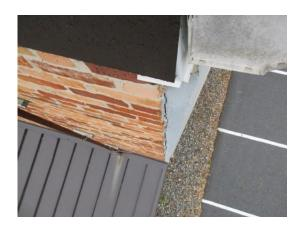
X.2 \$\$ Caulk or tar has been applied to trim over the exterior of some of the windows, usually an unprofessional attempt to remedy roof leakage. Request a qualified contractor to install professional repair (probably flashing). See related remarks below.
