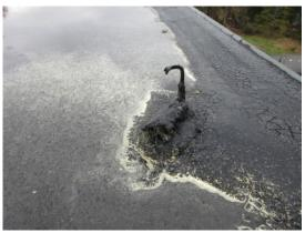
R.3 \$\$\$ Two sump pumps have been placed on this roof. If there has been leakage, this is not a professional repair.
