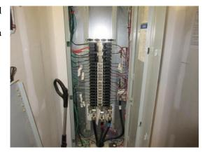
E.2 **SAFETY** \$ Hot and neutral wires are reversed at the water chiller receptacle.
