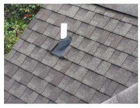
R.5 \$\$ A front left pipe (probably for the tankless water heater) lacks a boot. See related remarks in the Attic section.
