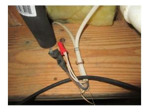
E.9 **SAFETY \$** Wires in a junction box at the left rear of the crawlspace are not properly terminated.
