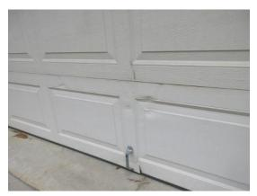
G.c The garage door has no weather stripping at the top and sides, typical for age. Repair as desired.
