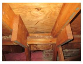
A.5 \$\$ There is an opening in the ceiling or between walls at the right of the HVAC equipment through which attic air spills next to uninsulated walls. This area should be covered/sealed with appropriate fire blocking material where applicable and insulated for improved energy efficiency.
