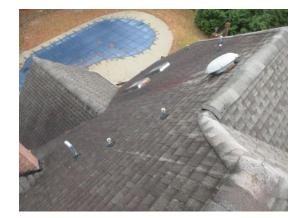
R.c The area where the valley intersects with the second level at the left of the front entrance wall is leak-prone due to design.Evidence of leakage was observed, as noted in the Crawlspace section.
