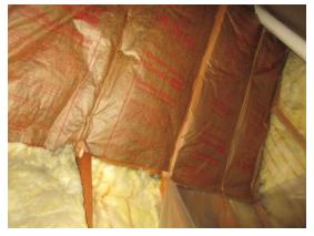
A.3 \$\$ Roof sheathing especially at the tankless water heater flue area is moisture stained. This area was wet when tested with an electronic moisture meter, indicating active leakage. See related remarks in the Roof section.
