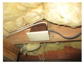
E.6 **SAFETY \$\$** Some cables entering the laundry electrical panel lack pull restraints (romex clamps).
